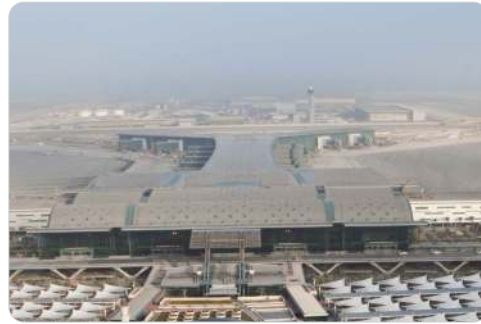
Roof of Doha Airport in Qatar. Picture courtesy of Hamad International Airport
