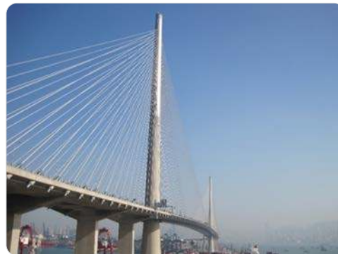
Stonecutter's bridge in Hong Kong. Picture courtesy of Outokumpu Oyj
