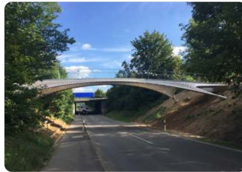
Footbridge of Trumpf, Ditzingen, Germany Picture courtesy of Schlaich Bergermann Partner
