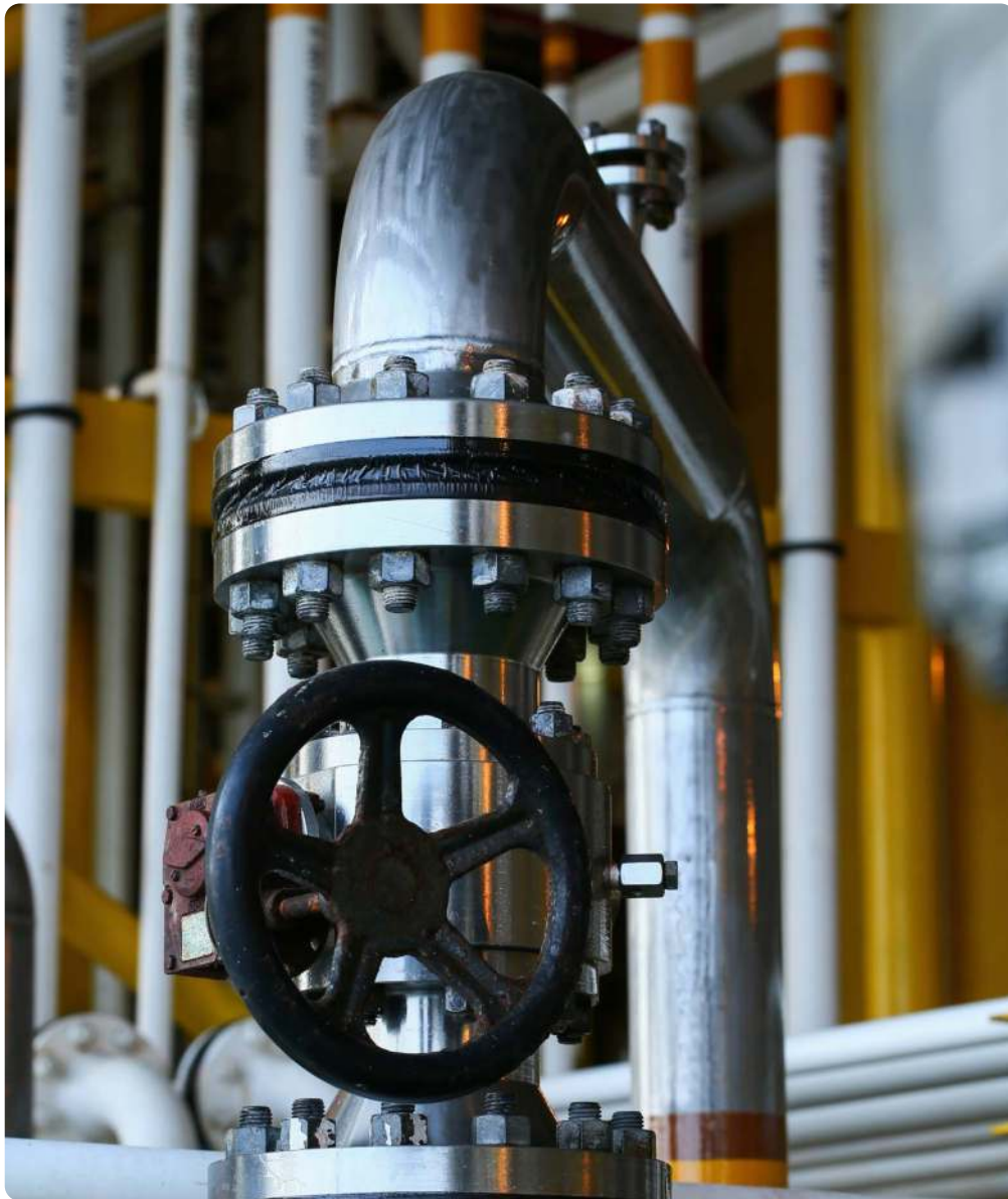
Duplex stainless steel manual valve in the oil and gas production process
