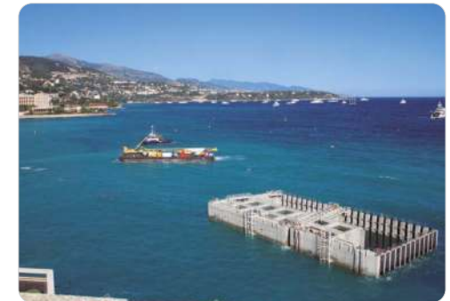
Monaco Extension on the sea Picture courtesy of Bouygues TP
