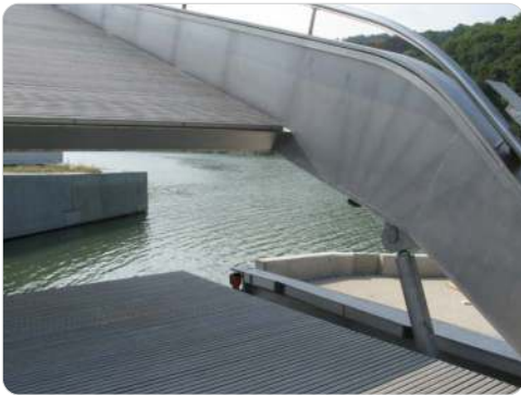
Bascule Pedestrian Bridge Picture courtesy of Industeel
