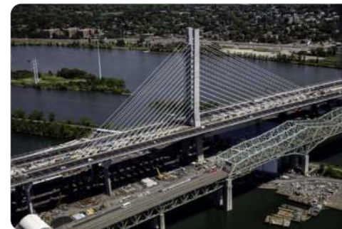
Champlain Bridge in Montreal, Canada. Picture courtesy of Infrastructure Canada
