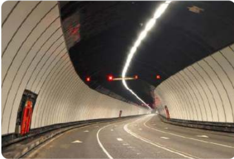
Lining of the Queensway tunnel in Liverpool Picture courtesy of Ancon Ltd
