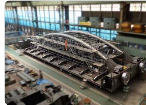
Kamihirai Floodgate in Japan Picture courtesy of NIPPON STEEL Stainless Steel Corporation
