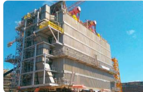
Blast wall Picture courtesy of Mech Tool Engineering
