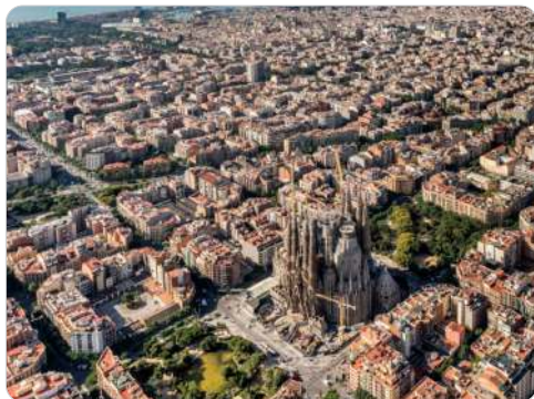
La Sagrada Familia by Antoni Gaudí in Barcelona. Picture courtesy of Outokumpu Oyj.
