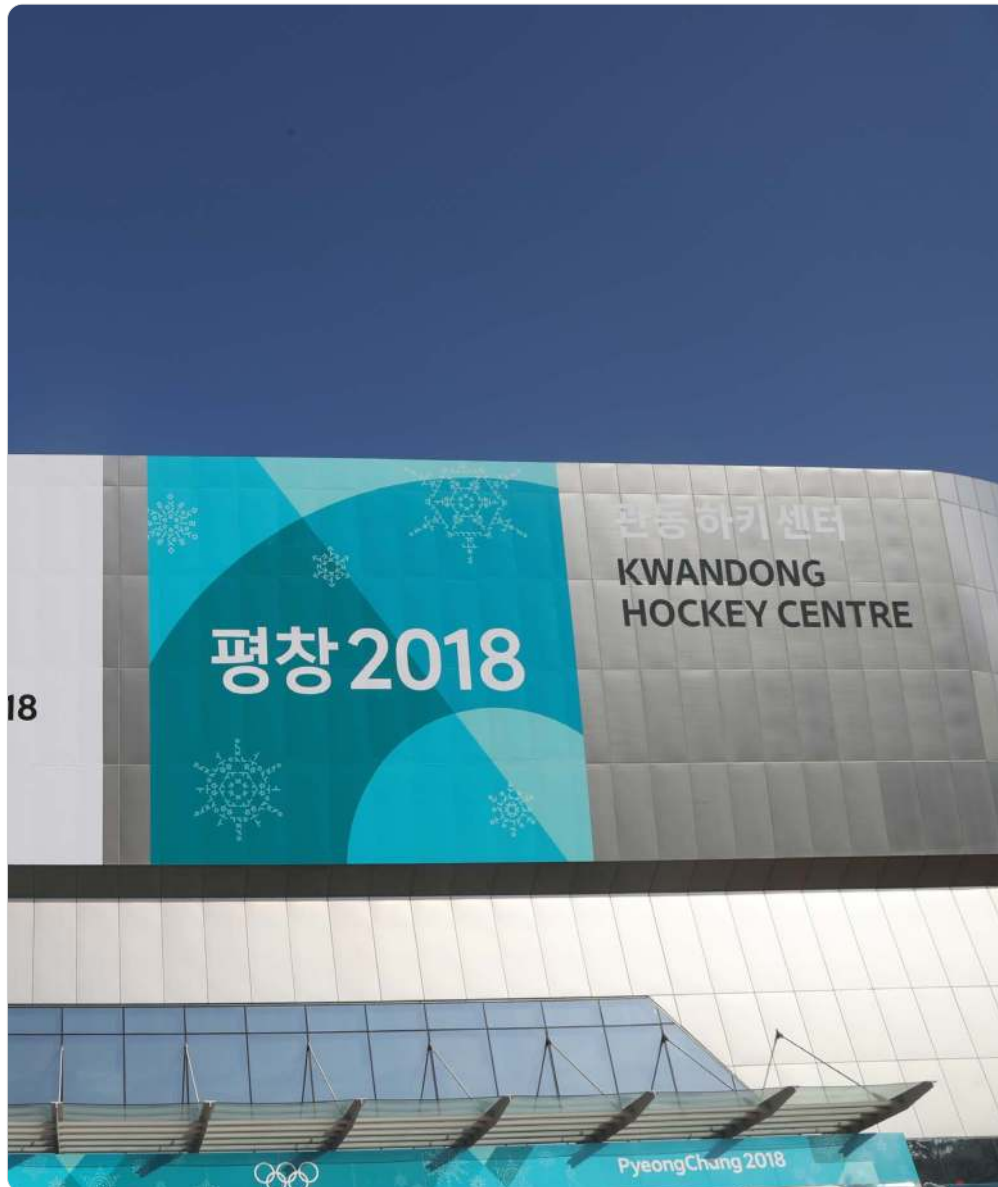
Detail of the Kwandong Ice Hockey Center in Korea, clad in lean duplex 329LD
