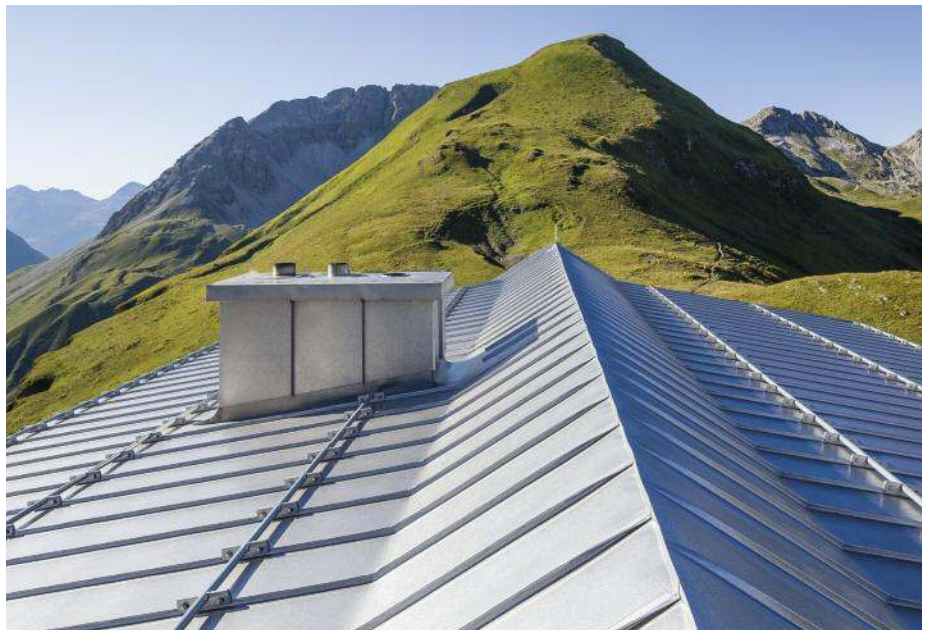
This stainless steel standing seam roof uses the double lock technique to provide a permanent seal in this harsh mountain environment, characterized by high winds, heavy snow loads and extreme temperatures. © Roofinox
