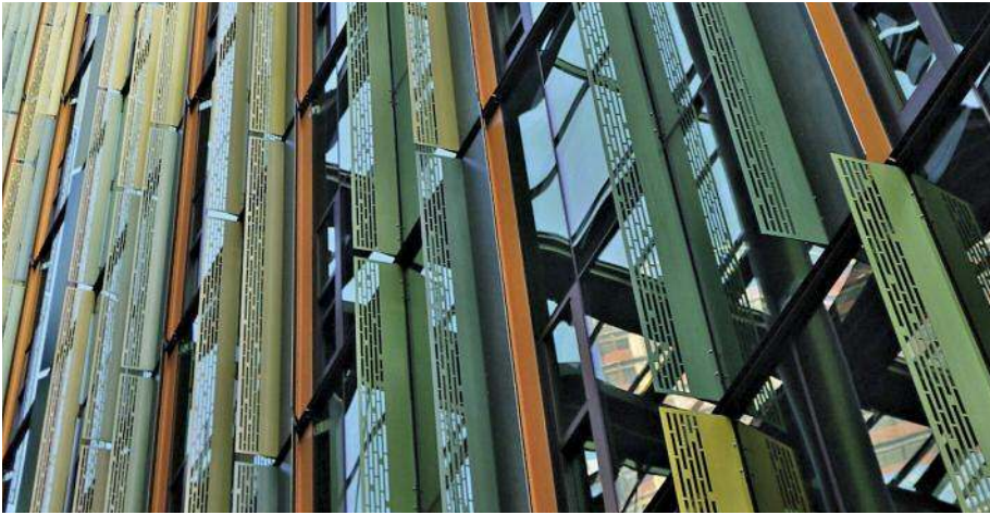
Electrochemically colored stainless steel fins (except orange) on the Doppler Building in Seattle. © IMO A
