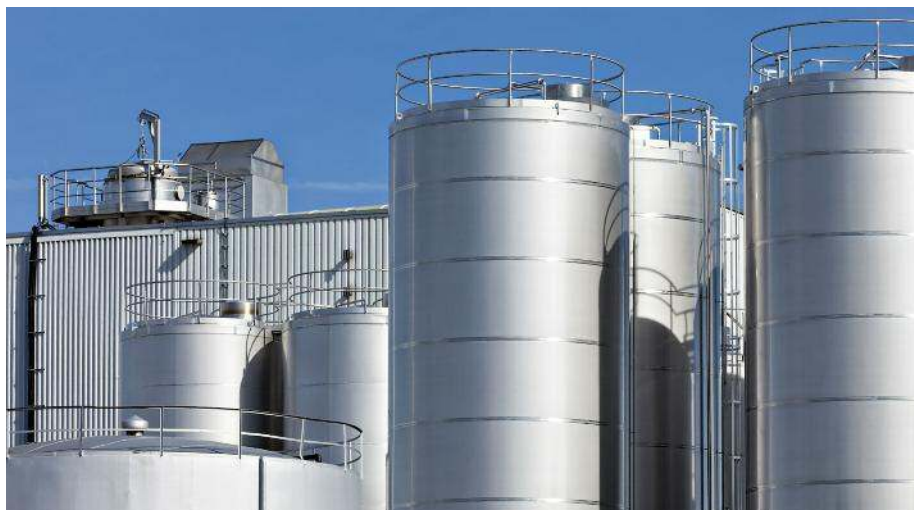
Welded stainless steel storage tanks in a dairy plant. © iStock.com/Bim
