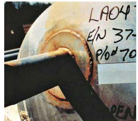
Carbon steel wire brushes used to clean stainless steel welds can produce discoloration and rust. © Outokumpu Stainless
