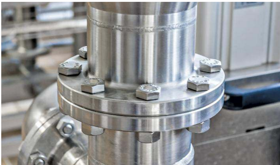
Bolted flange connection. © Super8/Shutterstock.com
