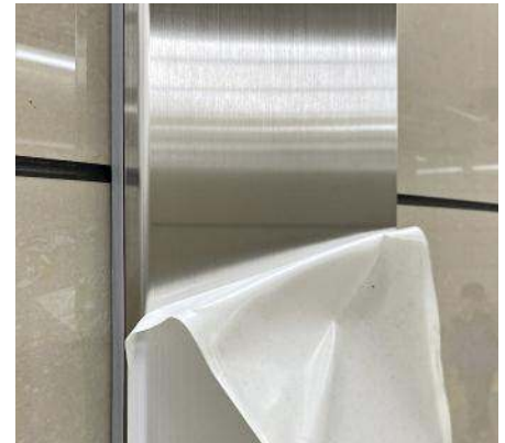
Strippable film protects the stainless steel surface finish from scratching and dirt during fabrication and transport. © IMO A
