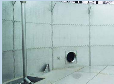
Inside views of a stainless steel fermenter
