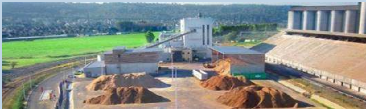
9 MW wood residue CHP plant (Rouen, France) which uses combustion to generate energy
