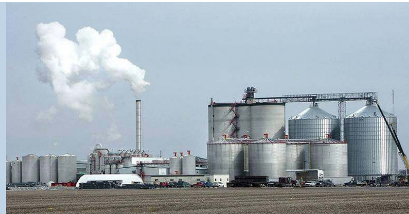
280 MW corn bioethanol plant (West Burlington, USA)
