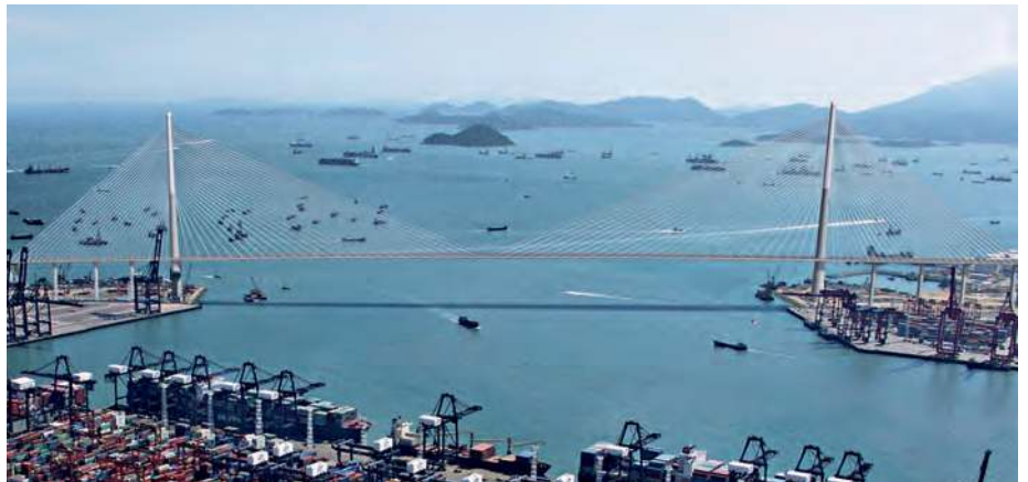
Stonecutters Bridge, Hong Kong. © Ove Arup & Partners
